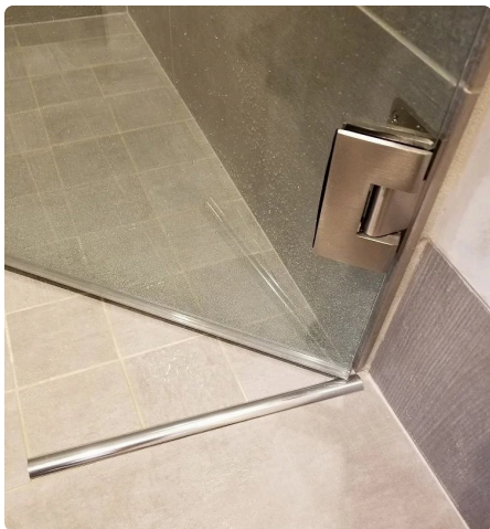
Water dam at a curbless shower opening. Photo: DT Glass, Oregon City, Oregon.
