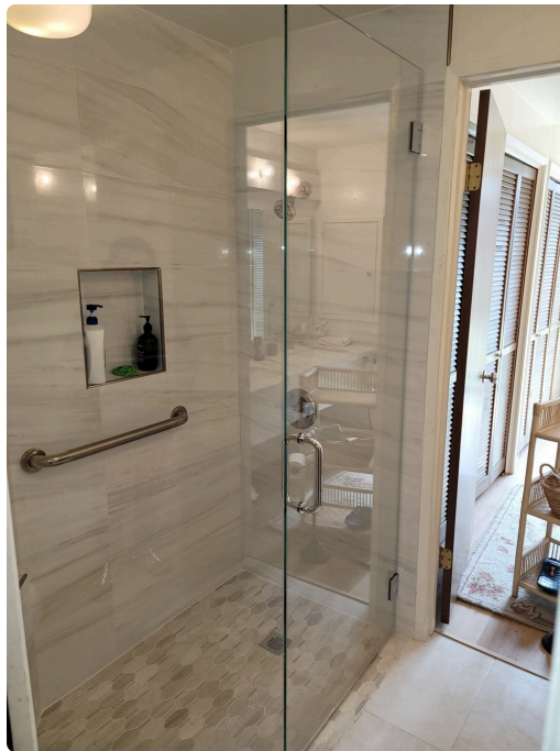
Curbless shower enclosure installed by Lincoln Shower Door. Photo: Lincoln Shower Door.
